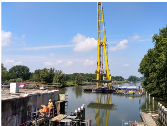
Figure 7. The lifting of the bridge deck.
