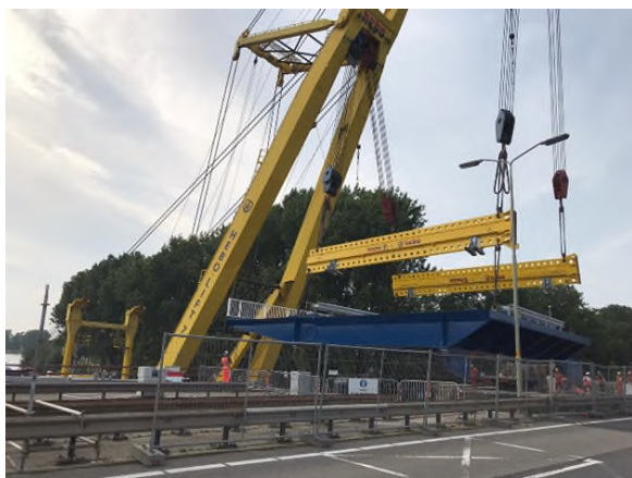
Figure 8. The lifting of the bridge deck.
