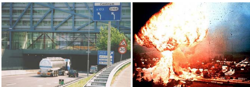
Figure 3. The transport of LPG (Liquefied Petroleum Gas) may cause an explosion, resulting in a fireball with an effect diameter of more than 300 m.
