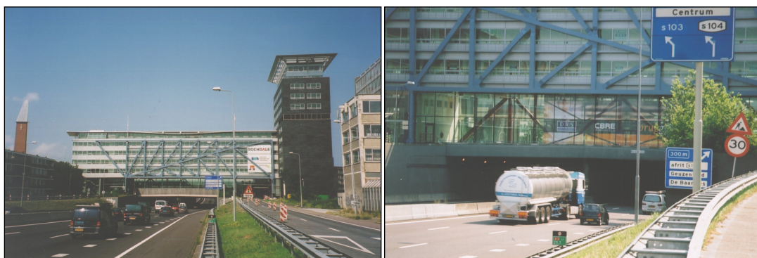
Figure 2: An impression of the Bos en Lommer Office buildings with transport of hazardous materials.
