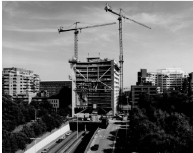
Figure 1: Construction of the Malie Tower in The Hague
