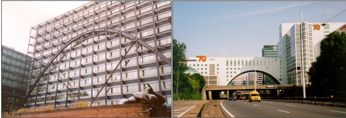
Figure 6.7: Examples of structural measures in buildings; Exchange House in London, UK (left) and the Haagse Poort in The Hague, The Netherlands (right).
