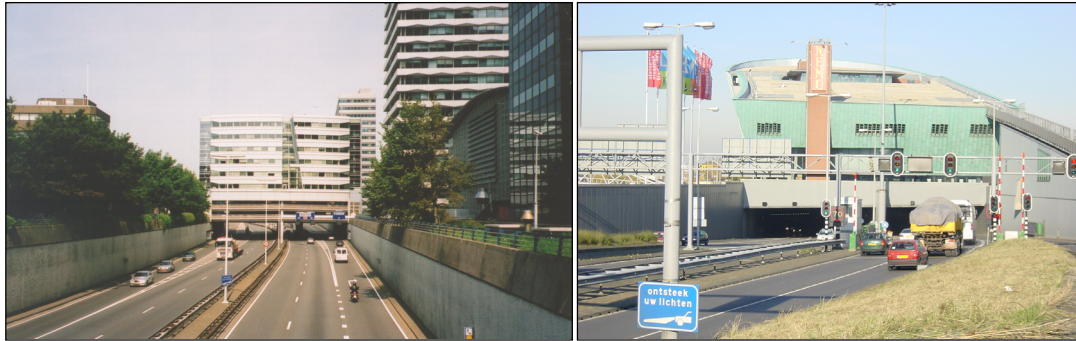
Figure 2.2: Buildings situated over the motorway in The Netherlands; the "Utrechtse Baan" in The Hague (left) and NewMetropolis in Amsterdam (right).
