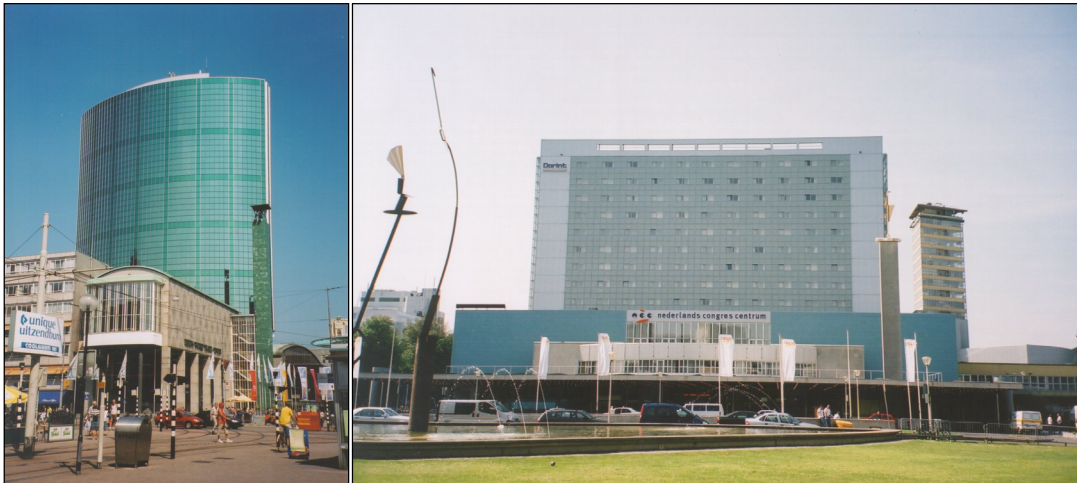
Figure 2.4: Buildings realised above existing buildings in The Netherlands; the World Trade Centre in Rotterdam (left) and Netherlands Congress Centre in The Hague (right).
