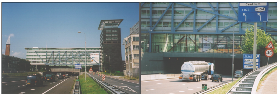
Figure 7.2: An impression of the Bos en Lommer Office buildings with transport of hazardous materials.
