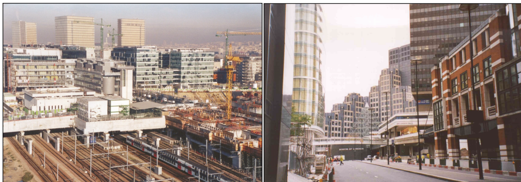
Figure 2.5: Multiple use of space projects: Building above railways in Rive Gauche, Paris, France (left) and building above roads in London, United Kingdom (right).
