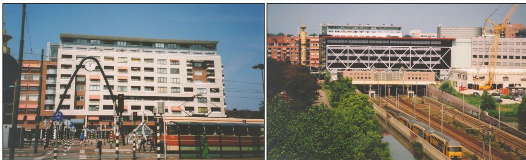
Figure 2.3: Railway station Rijswijk in The Netherlands covered by buildings; residential building (left) and an office building (right).
