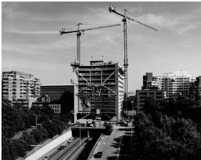
Figure 14. Construction of the Malie Tower in The Hague (The Netherlands).
