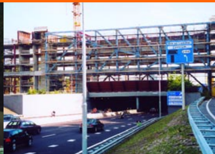
Overbouwing Ring A10 west.
