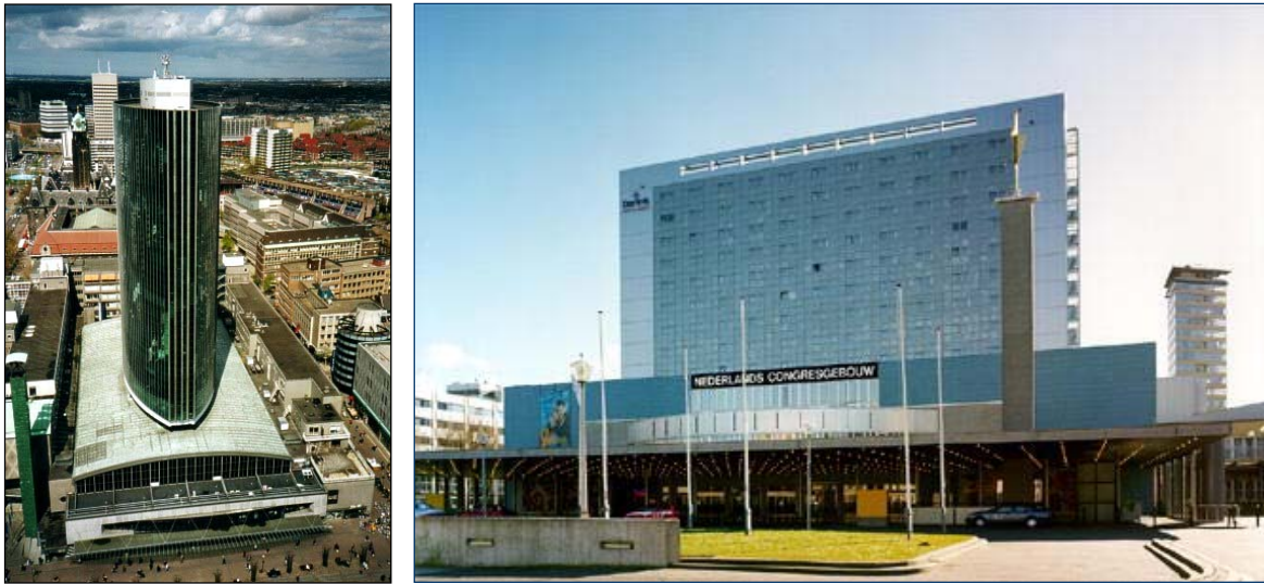
Figure 4: Buildings realised above existing buildings in The Netherlands; the World Trade Centre in Rotterdam (left) and Netherlands Congress Centre in The Hague (right).
