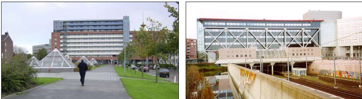
Figure 3: Railway station Rijswijk in The Netherlands covered by buildings; residential building (left) and an office building (right).
