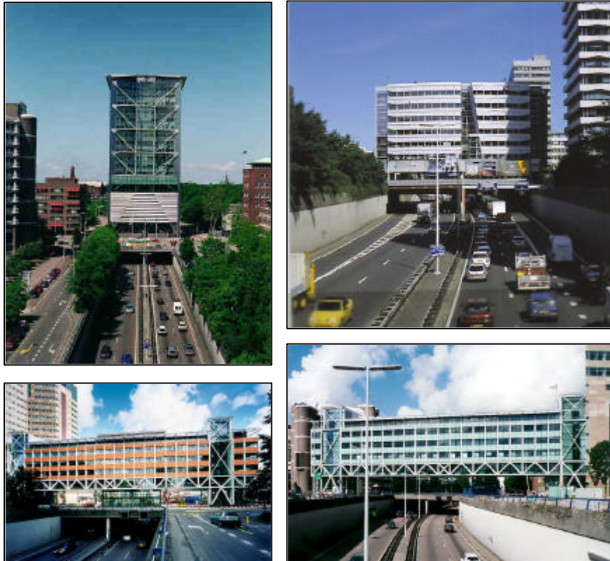
Figure 1: Buildings realised above a motorway "The Utrechtse Baan" in The Hague, The Netherlands.
