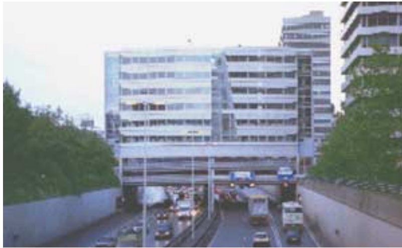
Figure 3: The Equinox building in the Hague was cost-effective as it used the existing motorway trough as a foundation.
