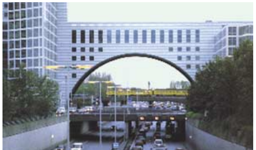
Figure 2: The Haagse Poort office building constructed above the Utrechtse Baan motorway while still in use.
